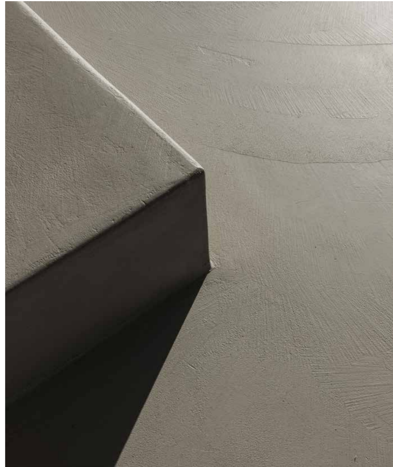
Private House - Mantova GeoOutdoor
